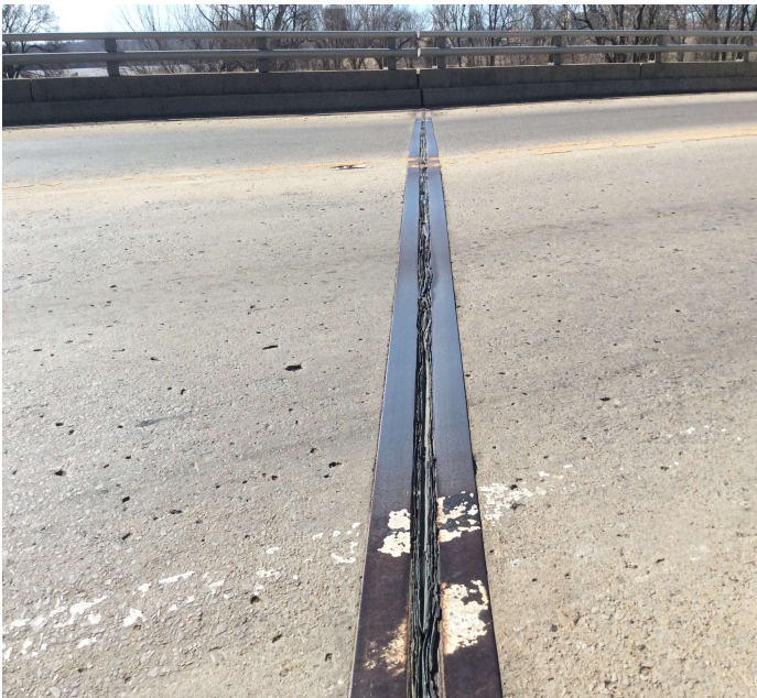
PHOTO 1 Description The compression deck joint seals have rips, tears and leak on the bent caps.
