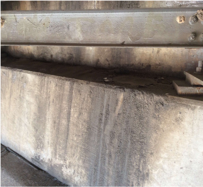
PHOTO 1 Description Dirt accumulation on Bents # 1 & 4 cap.
