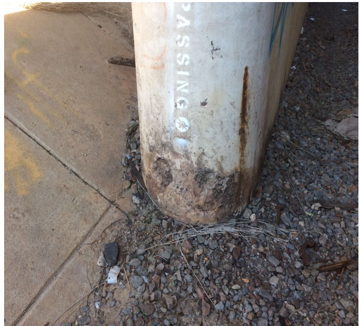
PHOTO 2 Description Spalling at the West column base is approx. 1" deep and 14" tall.
