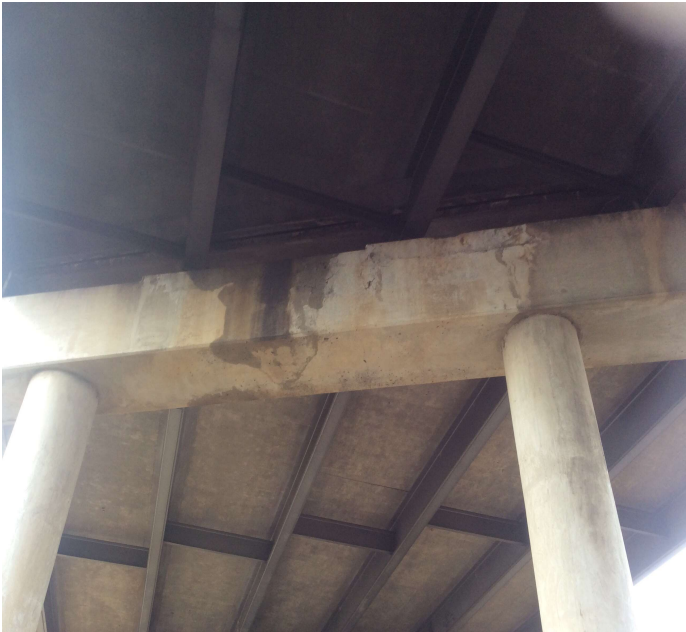
PHOTO 1 Description Concrete delamination with exposed reinforcing steel on the caps
