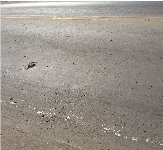
PHOTO 1 Description Minor sealable cracks on the driving surface of the deck.
