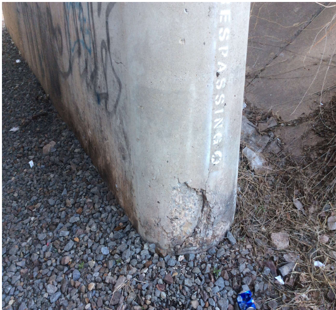
PHOTO 1 Description Spalling at the East column base is approx. 2" deep and 12" tall. Sounding indicates that there is 12" of additional delamination of concrete above the spall.
