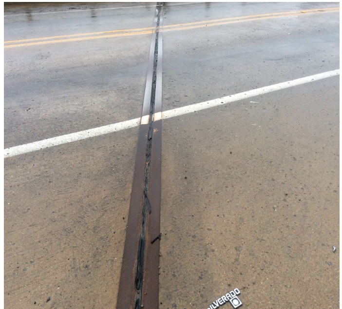
PHOTO 2 Description Typical compression joint seals.
